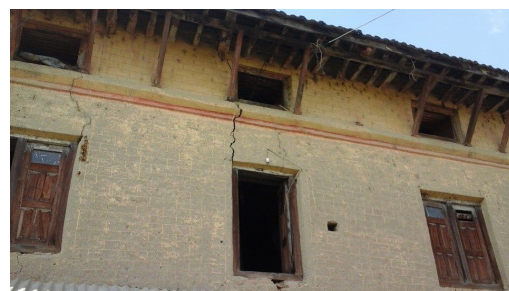
Structural damage to our house in earthquakes
